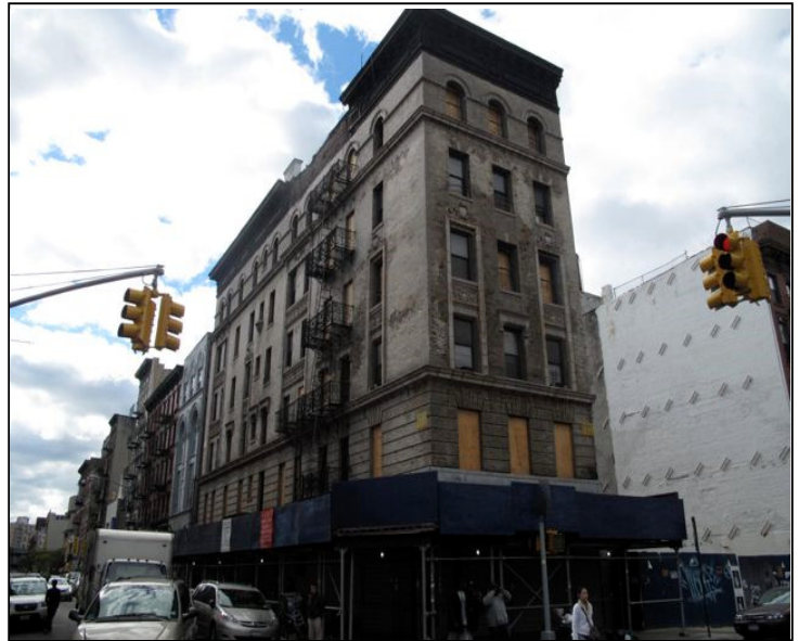
Picture of 289 Grand St. building as it stands today. It is the only damaged building to survive the April 11, 2010 fire.
